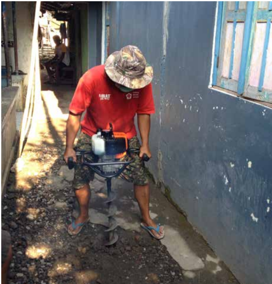
CBAT members are making biopori hole using a drilling machine to make it faster.
