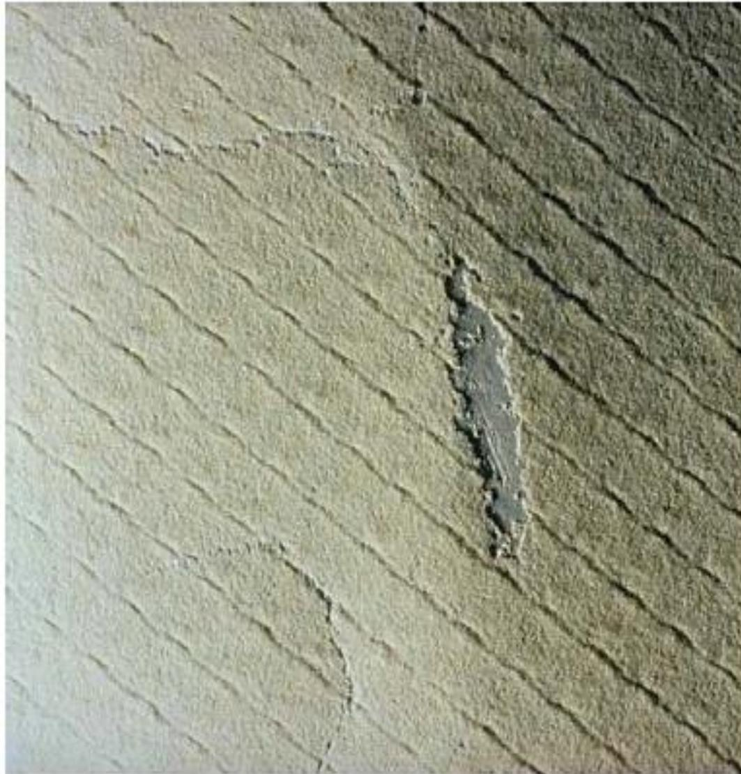
Figure 8.10 Picture of damaged fiberglass shell
