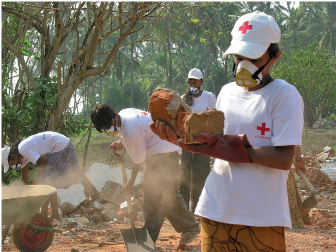
Volunteers clearing debris left by the destruction of homes in Beruwala, Sri Lanka. The clean up continued for months after the waves had hit. Photo: Lena Eskeland / IFRC
