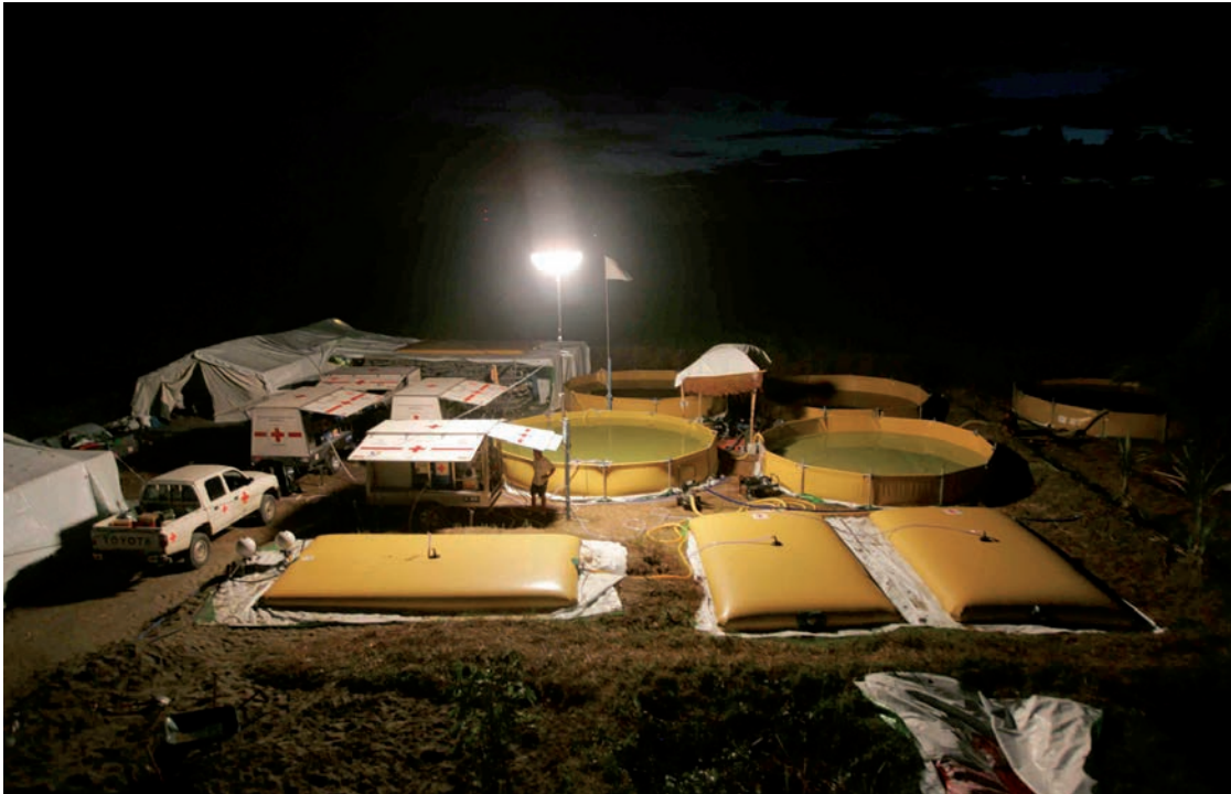
Water and sanitation ERU operated by the Spanish Red Cross in Indonesia, just two weeks after the disaster struck. By 28 January, it had provided more than four million litres of save water. Photo: IFRC
