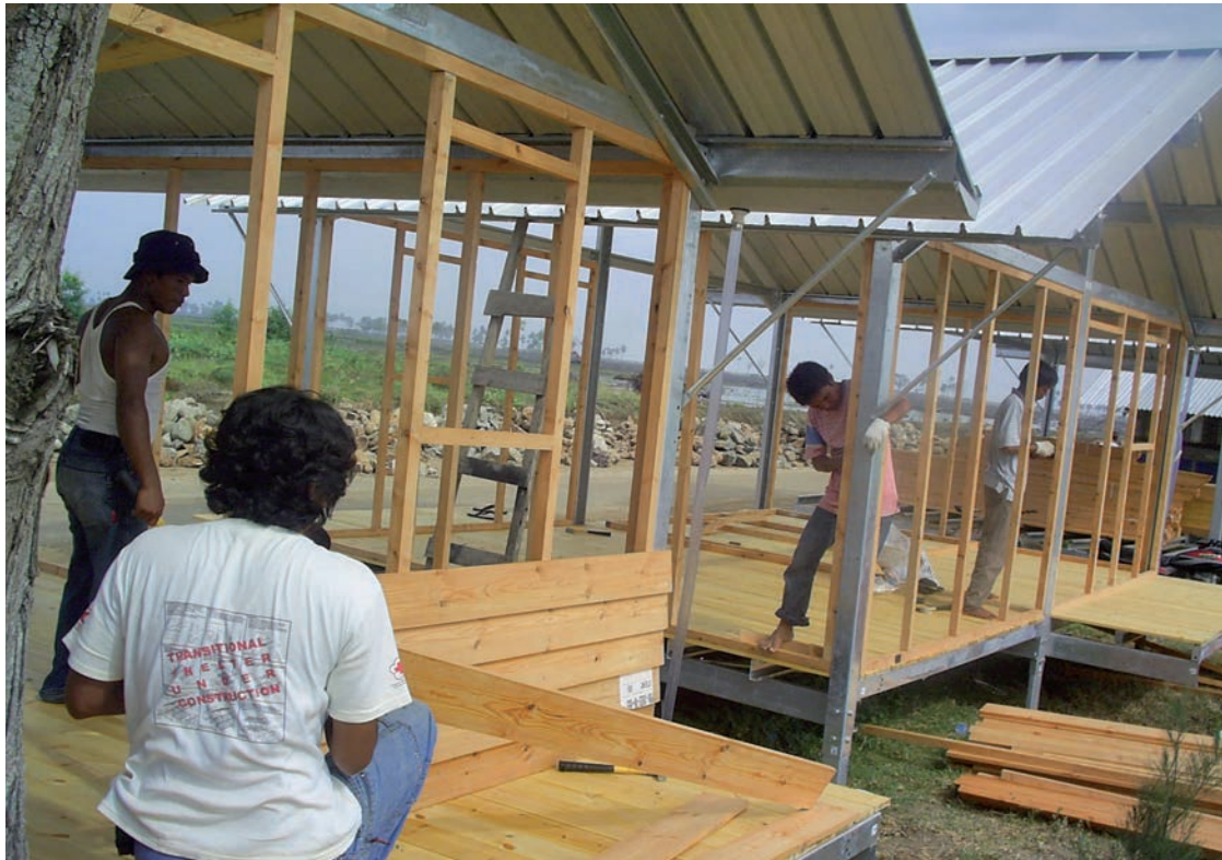
19,923 prefabricated temporary shelters were constructed in Indonesia following the tsunami. These material for shelters was shipped from overseas, helping to prevent illegal logging and protect the already damaged environment. Photo: IFRC
