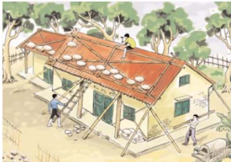
Picture 17 Reinforcing houses before typhoons
