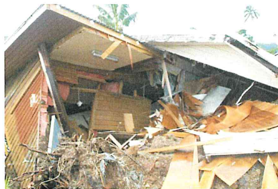
Landslide in Qamea, January 2017
