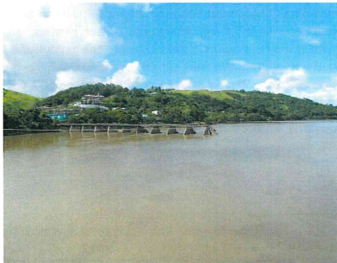
Sigatoka Bridge, January 2009
