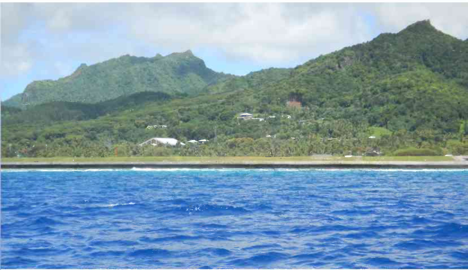
Seawall, Nikao, Rarotonga
