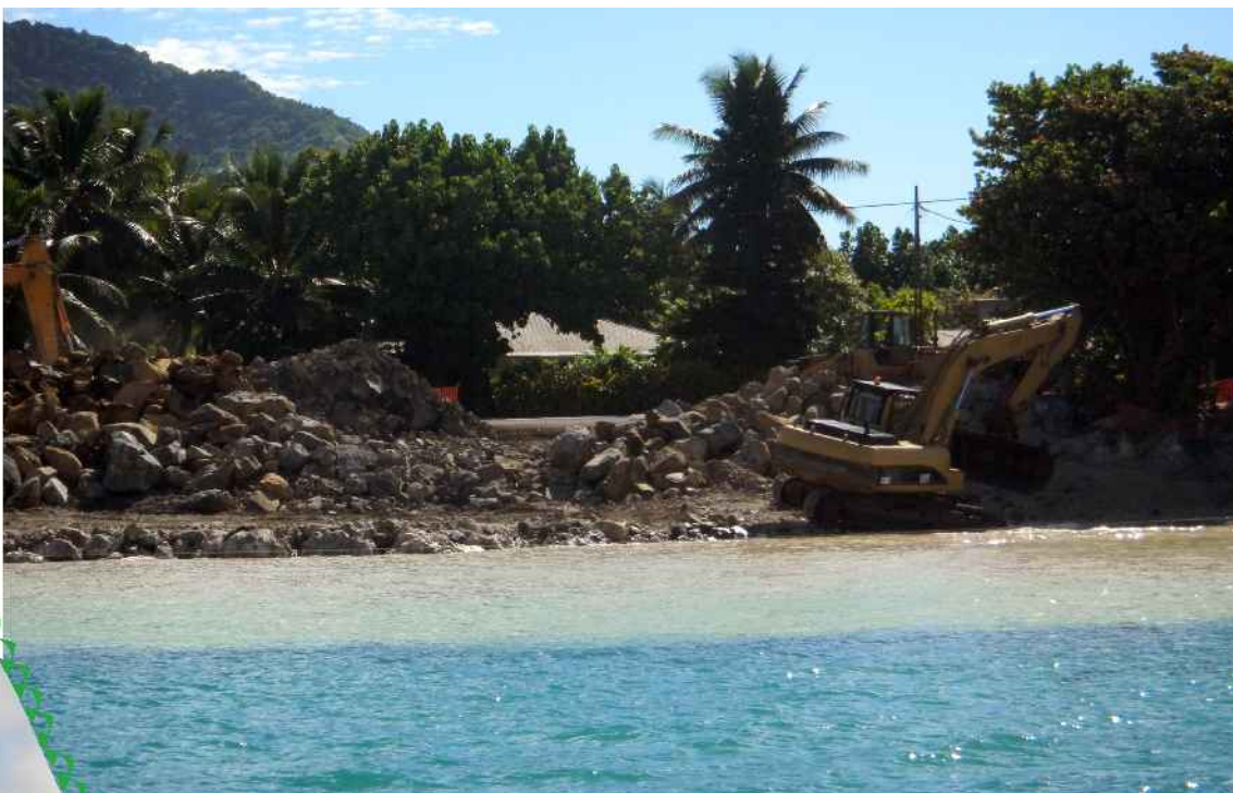
Harbour Construction, Avatiu, Rarotonga
