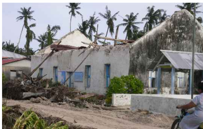
Damaged building in Pukapuka after TC Sally 2005
