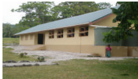
EU project built classroom– permanent
