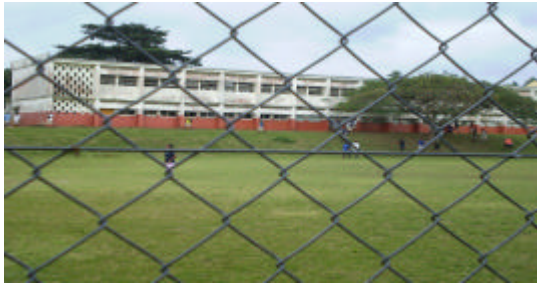
Another section of Lycee School is a double classroom Is an old building that is not safe during earthquake..
