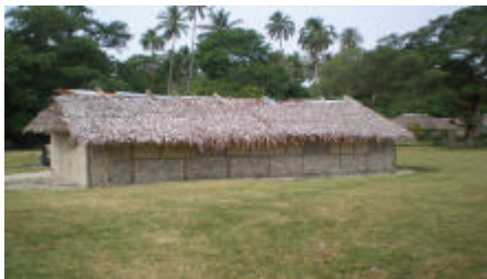
Stone local built classroom Malo English school
