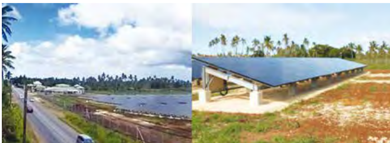
Figure 8.1 Solar Power Array built with JICA support as part of Tonga Energy Roadmap (credit: JICA) 92
