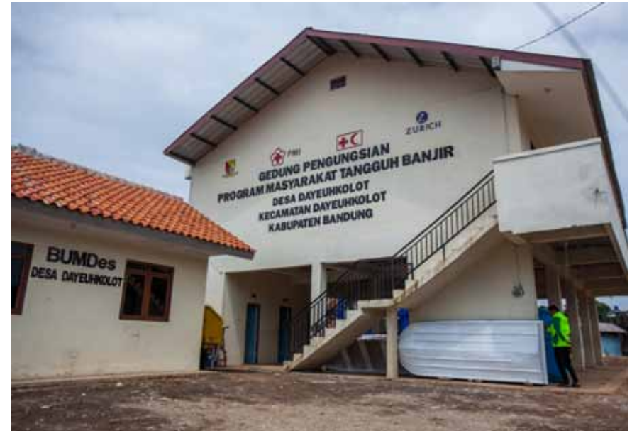
Evacuation building, supported by CFR program in Dayeuhkolot Village.
