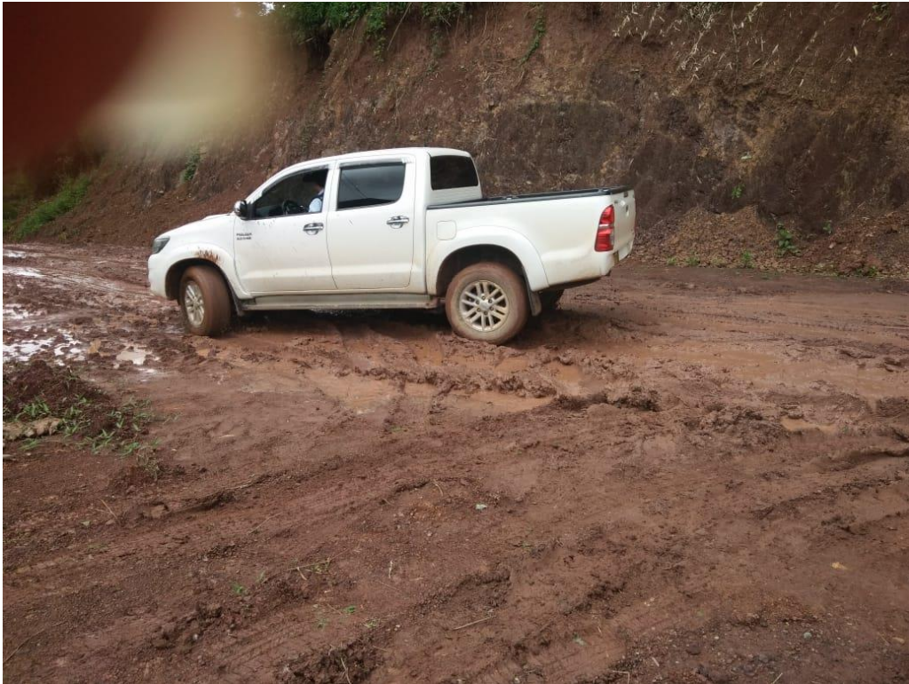
Road condition in Baeng district during the implementation of this activity.
