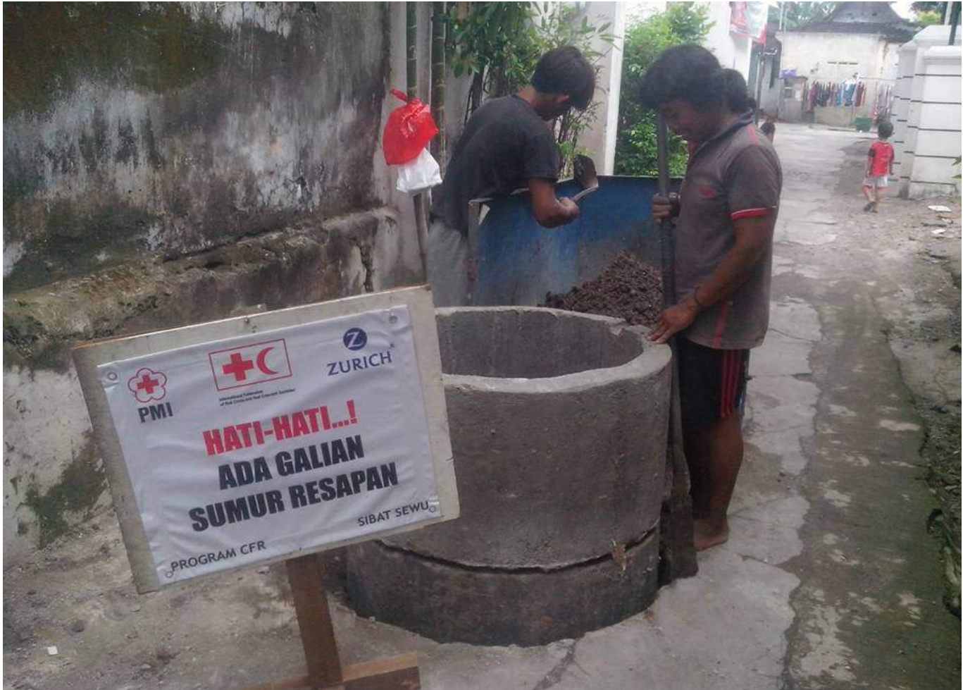
The team members of Sewu Village CBAT, Surakarta, are preparing a concrete ring as a material for making absorption wells.
