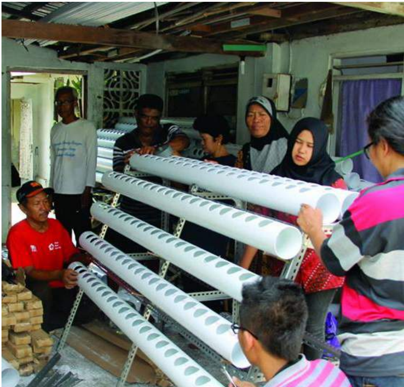
CBAT members of Sewu Village are installing the hydroponic garden of plastic and iron pipe materials. Photo: PMI
