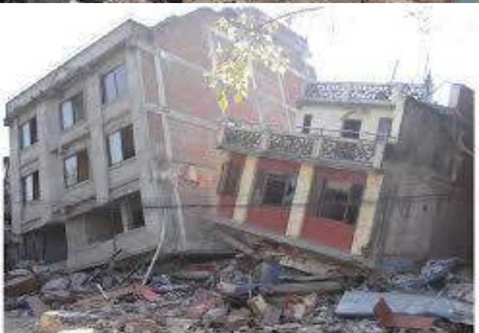
Collapse of RC frame buildings in Kathmandu
