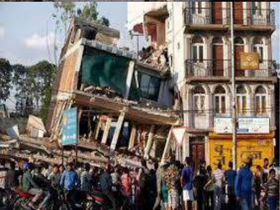
Collapse of RC frame buildings in Kathmandu
