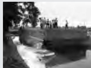
10. DEWATS intensive decentralized treatment plant
