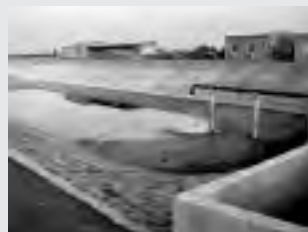
9. Waste stabilization pond
