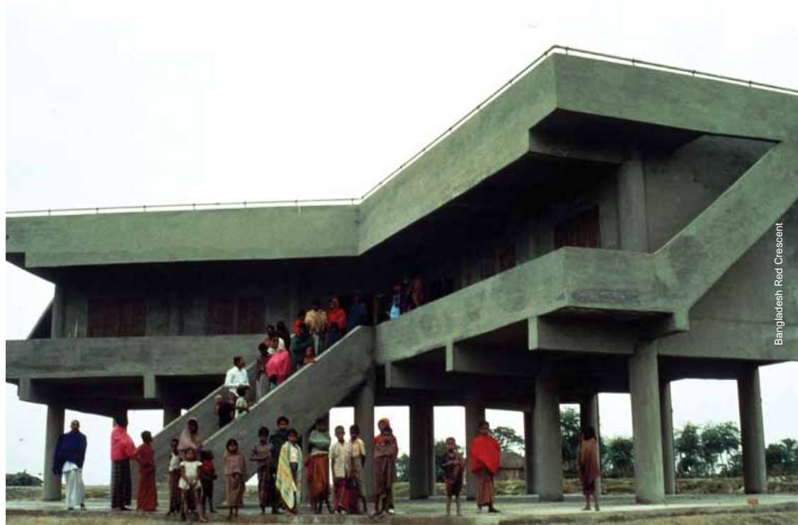
A cyclone shelter in Bangladesh which has helped save thousands of lives
