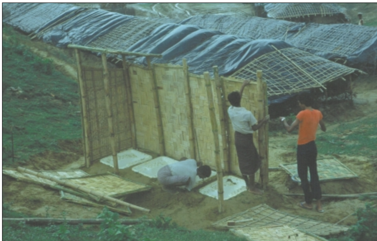
Borehole latrines nearing completion, Bangladesh
