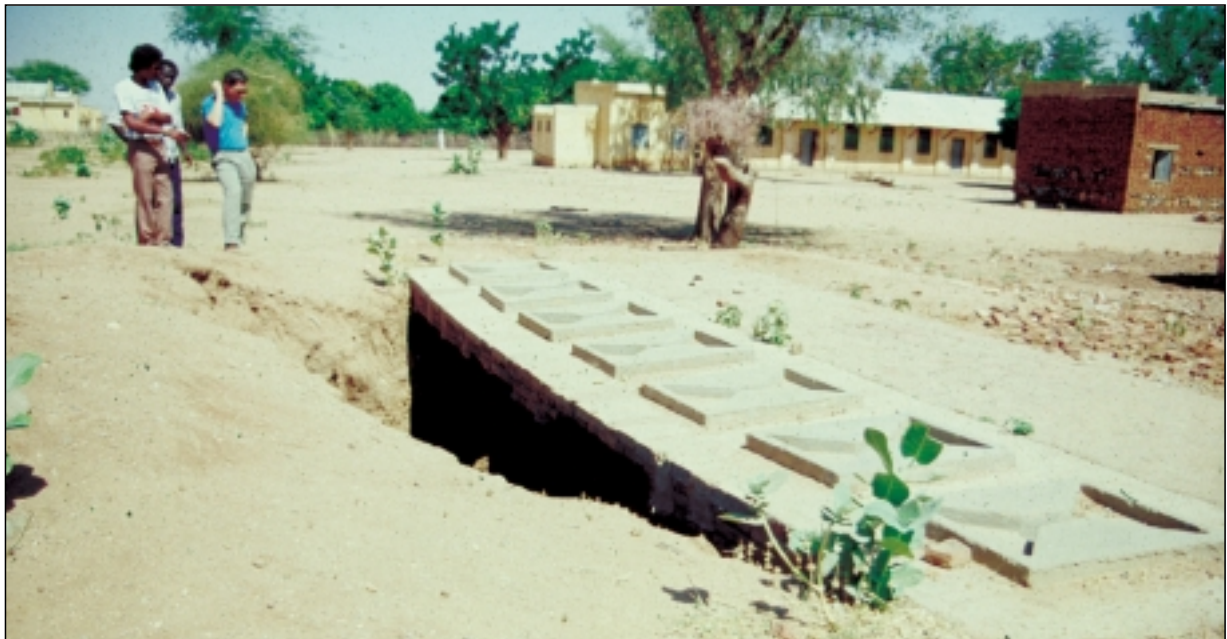
Failed unlined trench latrines, Sudan
