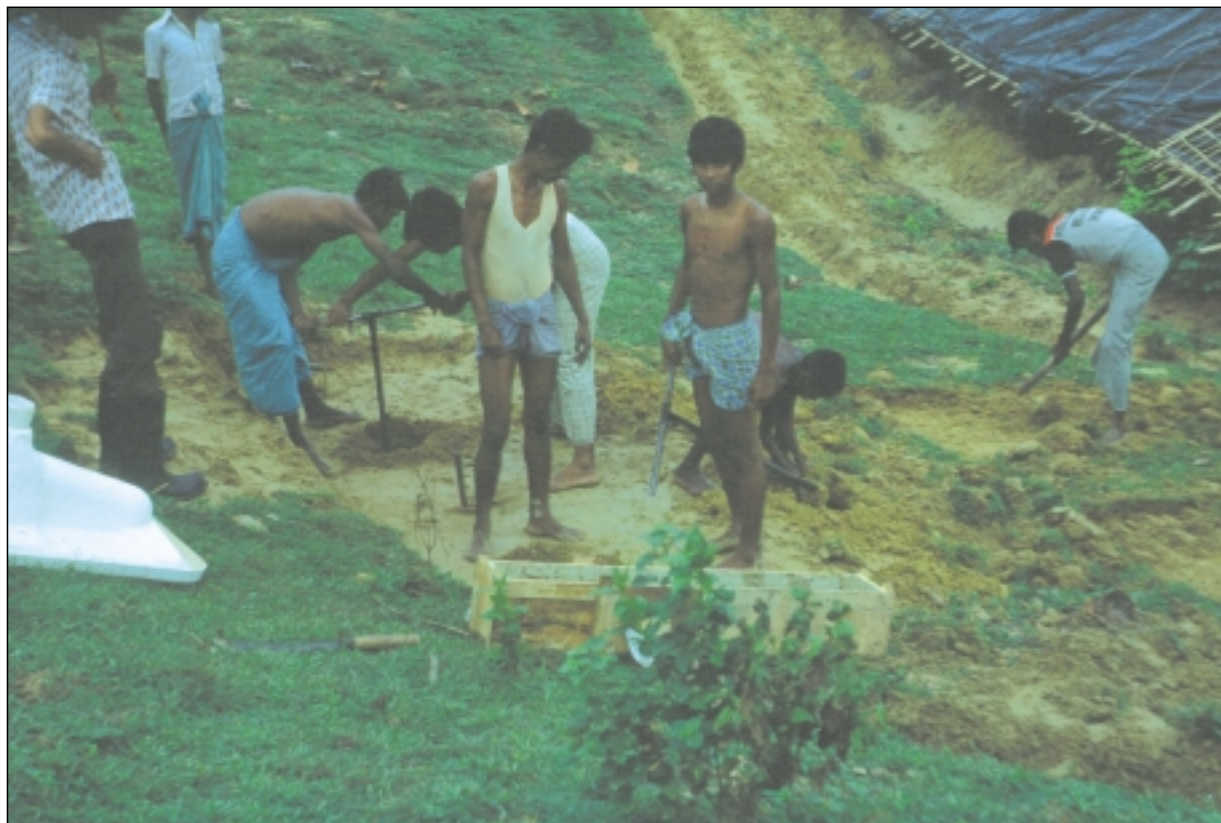
Drilling boreholes for latrines, Bangladesh
