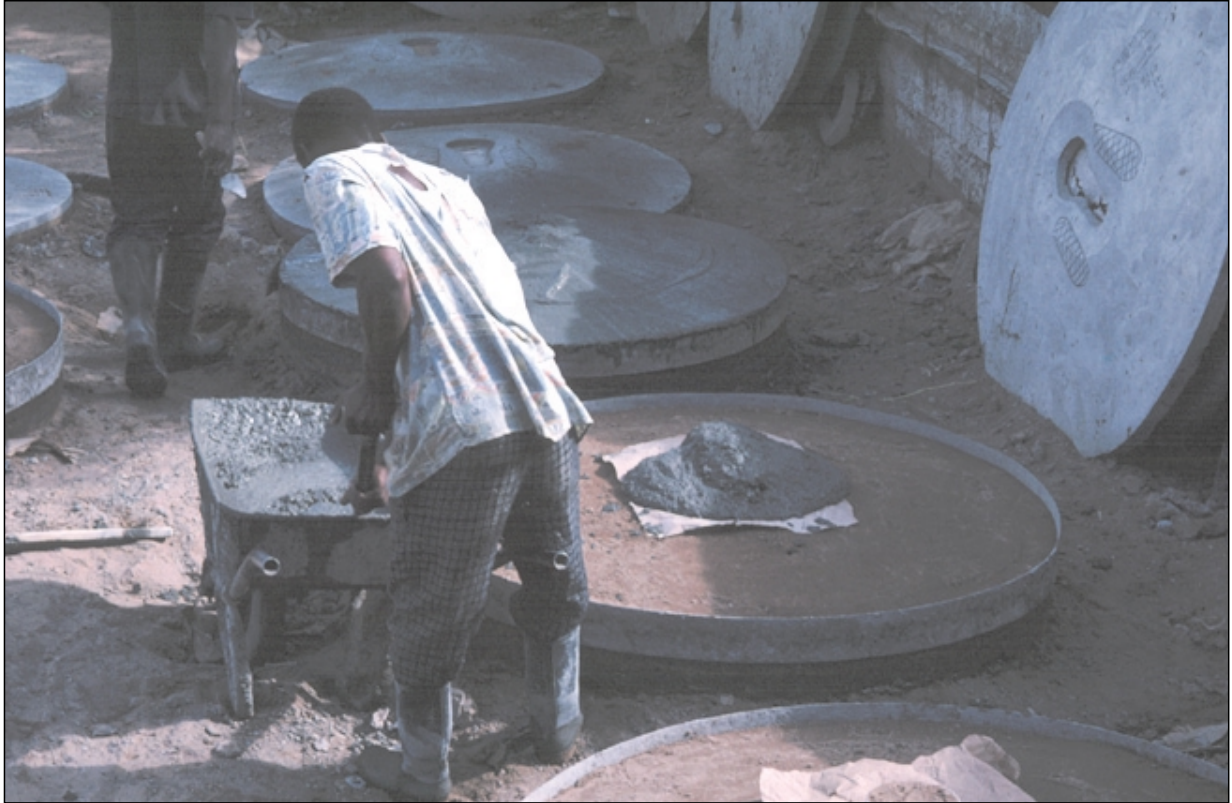
Producing latrine slabs in Mozambique
