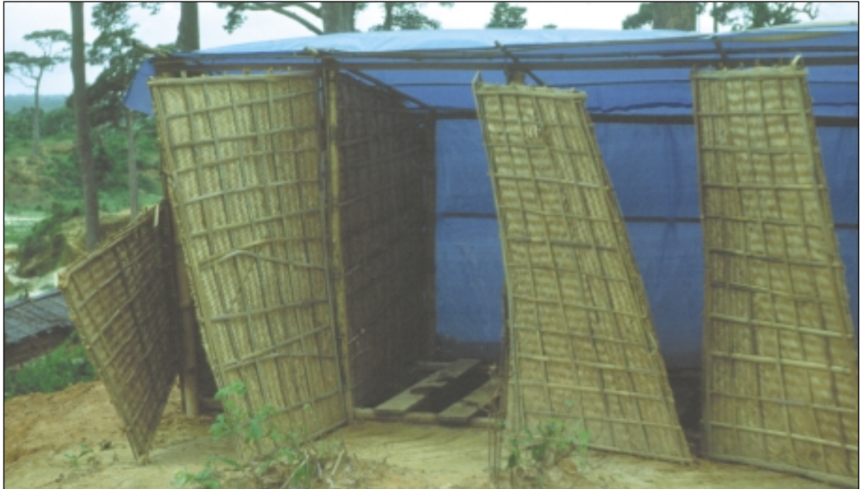
Simple trench latrines, Bangladesh
