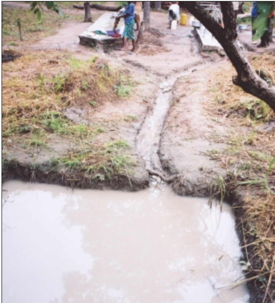
Poorly designed soakpit, Tanzania
