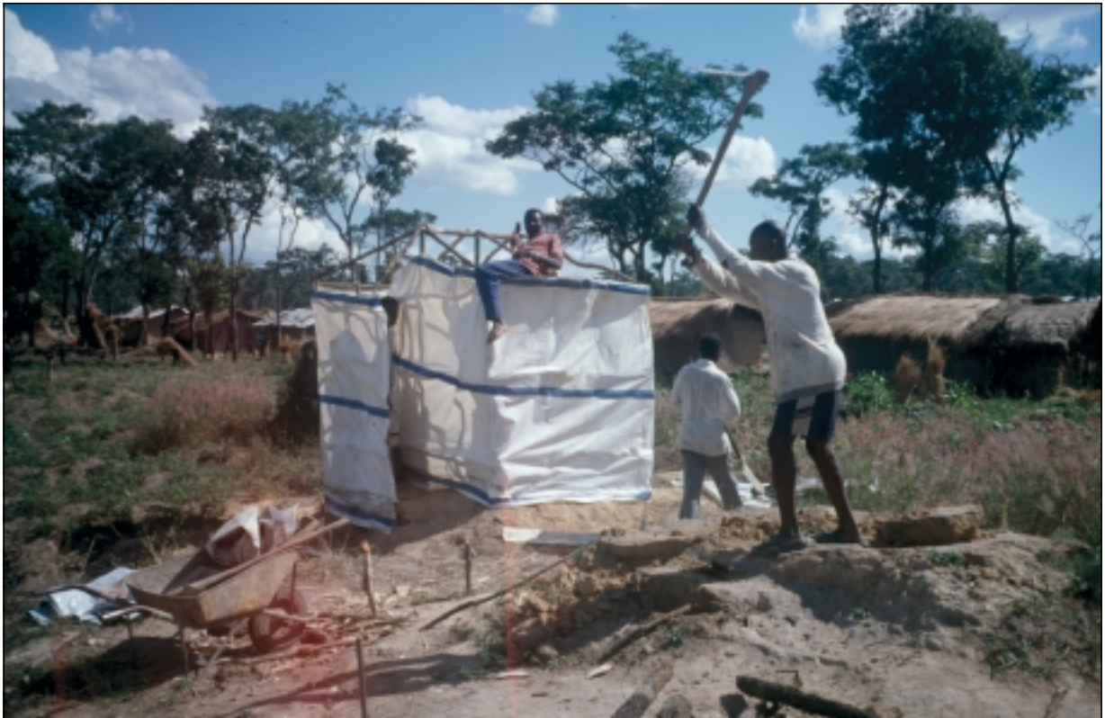
Pit latrine construction
