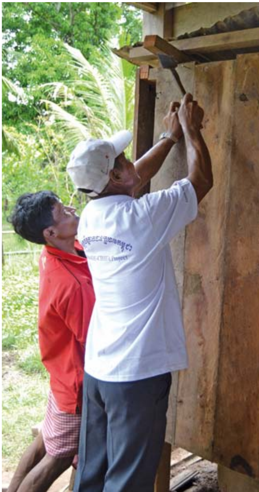
The National Society is assisting families to construct latrines. As a result of increased access to latrines and awareness raising activities led by volunteers, the percentage of people defecating in the open has gone down from 53 per cent to 8 per cent. Jessica Sallabank/IFRC
